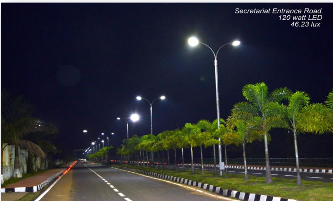
Airport Road near Army cantonment after LED installation
